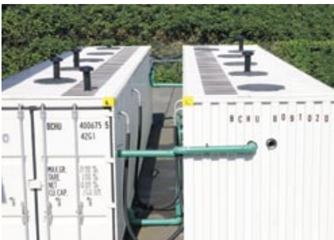
Pic 1: 40' treatment plant for 160 man oil exploration camp in Siberia
